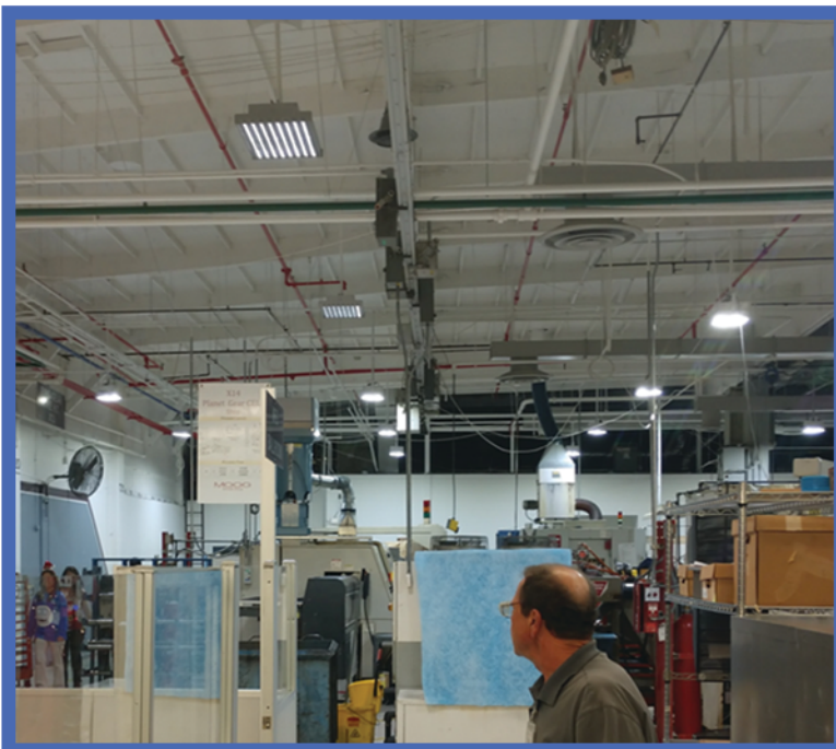
VHB3 fixtures on the left at about 18' Customer installed some UFO fixtures and they are total glare bombs - Pictured on the right
